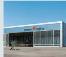
Ameco A380 Hangar Beijing, China
