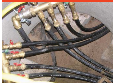
Fig. A.4.1-8 Brine distributor for geothermal probes
