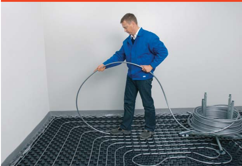
Fig. D.2.2-6 Area heating systems
