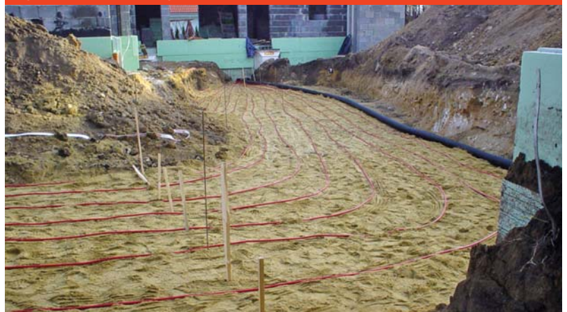
Fig. A.4.1-2 Heat source – geothermal collector
