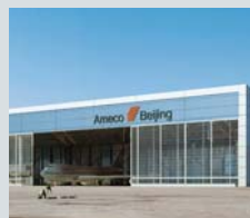
Ameco A380 Hangar Beijing, China
