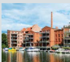
Studio flats, Brandenburg, Germany
